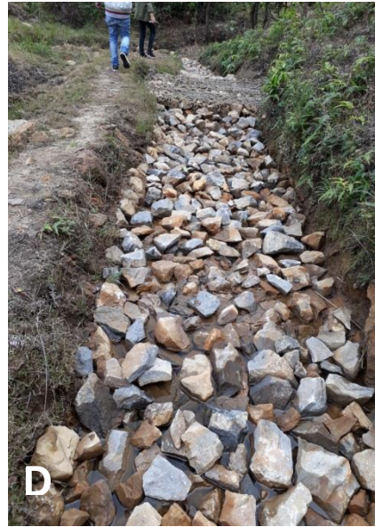
A. Photograph showing aerial view of Moolawar Streams (Streams A and B); B. Diagrammatic representation of Open Limestone Channel (OLC); C & D. View of Open Limestone Channels constructed on Moolawar Streams at Mukhialong Village, East Jaintia Hills District, Meghalaya
